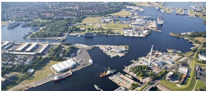
Access to key energy hub Wilhelmshaven, Germany
