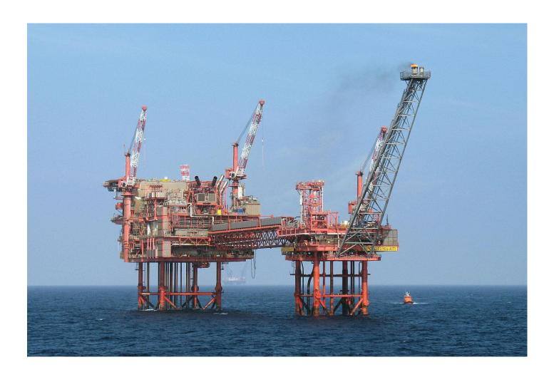
**North Everest** is a combined wellhead/production/quarters platform, producing gas and condensate from the North Everest field. The installation also processes gas and condensate from the South Everest subsea wellheads, located some 7.1km south of the North Everest production platform and Everest East Expansion (EEE) wells, located approximately 6.8km North East of the installation.
